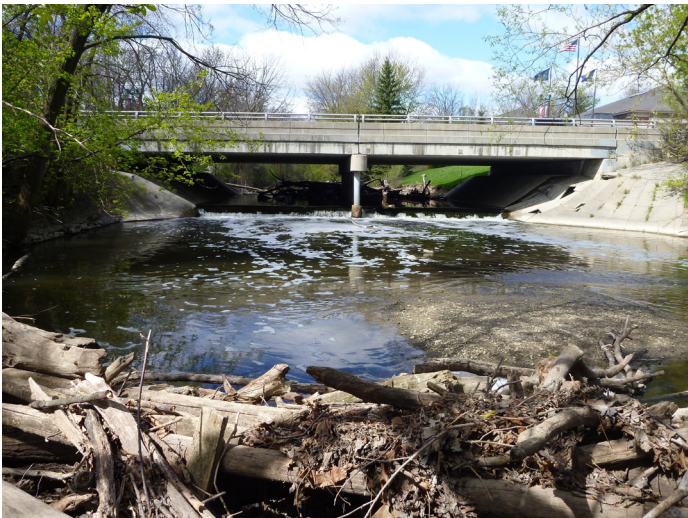
The Wayne Road dam before removal (left) and after removal (below left), and the bankfull benches (below).
